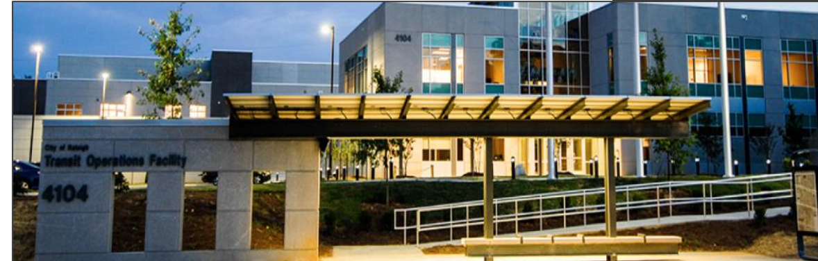
Current GoRaleigh O&M Facility in Raleigh, NC
